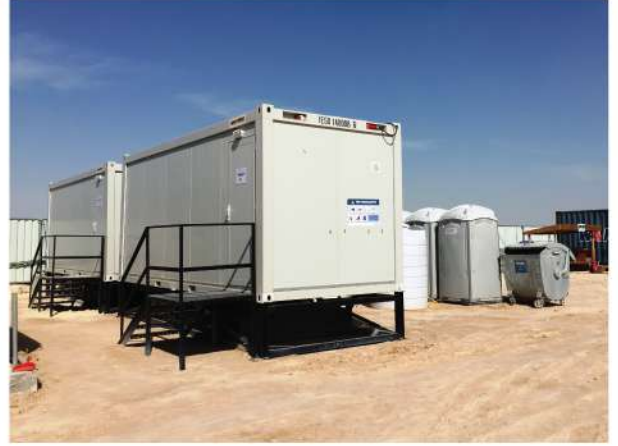
SHP Work site
